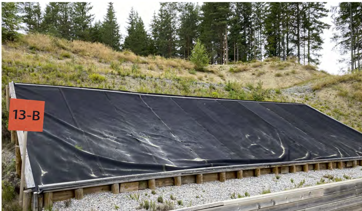
Figure 9 Range 13B at Sessvollmoen is a sand trap with a rubber sheet cover.
