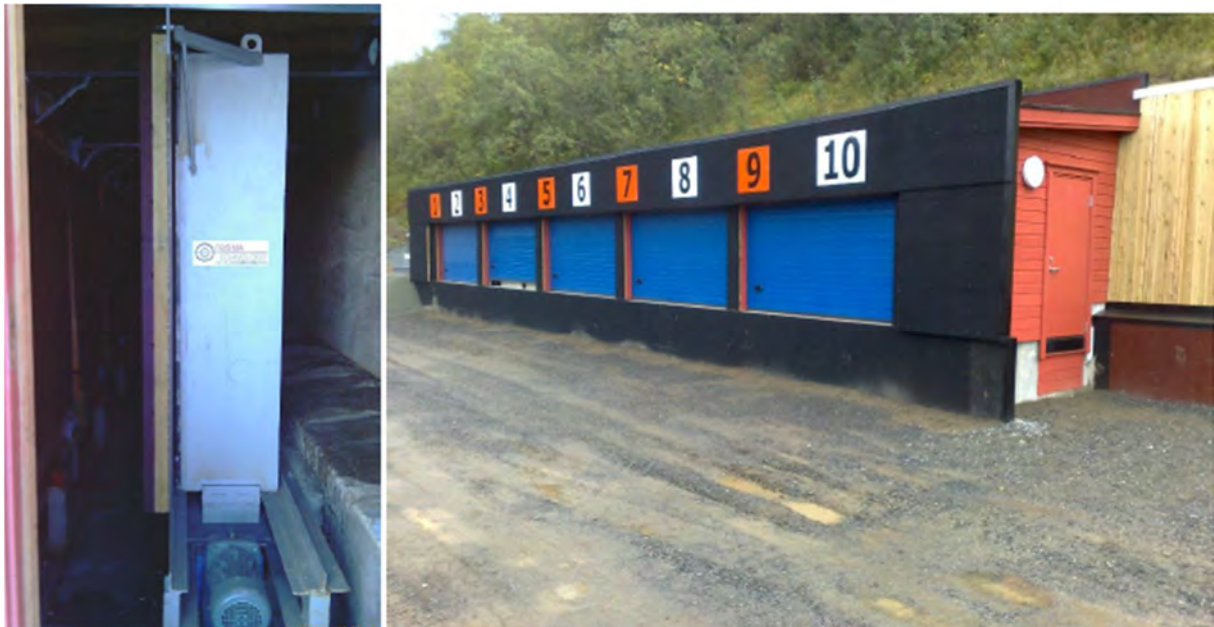
Figure 20 Lamella bullet trap, Camp Trondenes, with a conveying screw in the bottom to remove bullet fragments. (Forsvarsbygg, Håndbok for skyte- og øvingsfelt 2020 - 2022, 2020)
