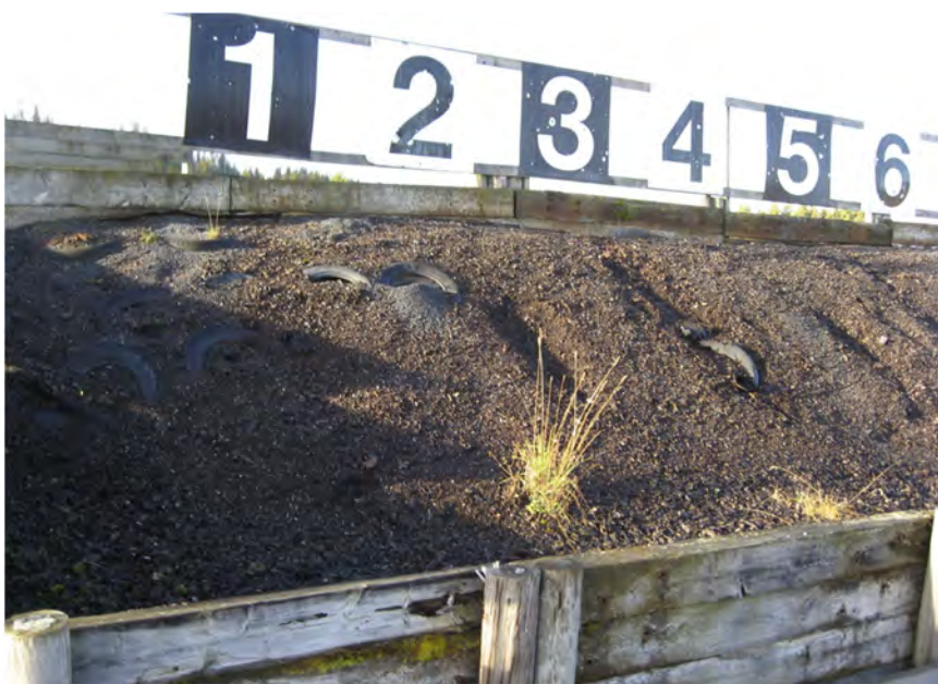
Figure 8 Close-up of a bullet trap with a box built of wooden poles and wooden beams to keep the soil/sand in the bullet trap
