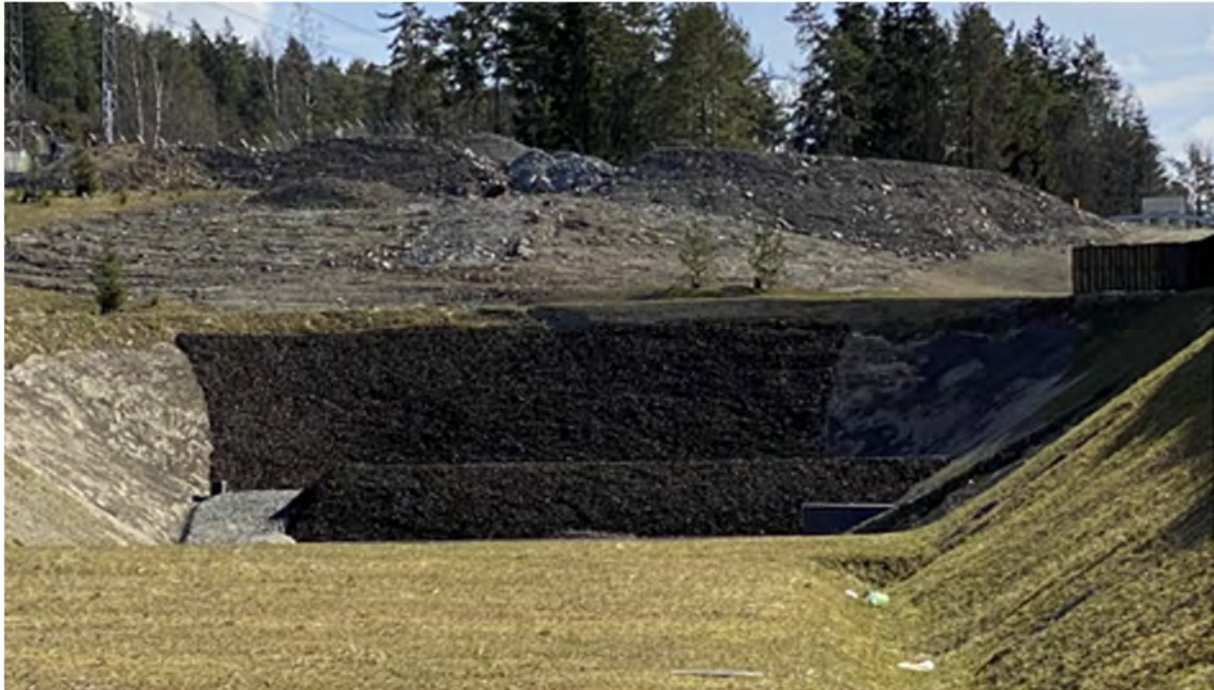
Figure 14 Target mound and bullet trap made of tyre chips, seen from the firing point
