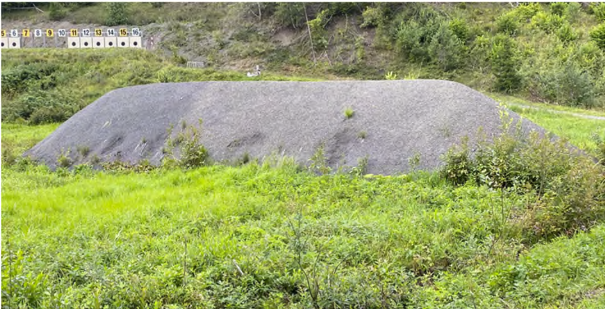
Figure 3 Bullet trap as a free-standing berm, in this case for Stang and field rapid shooting targets
