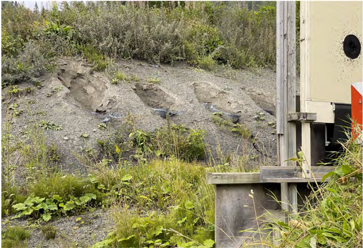
Figure 5 Example of old tyres used in bullet traps in an effort to stabilise mass
