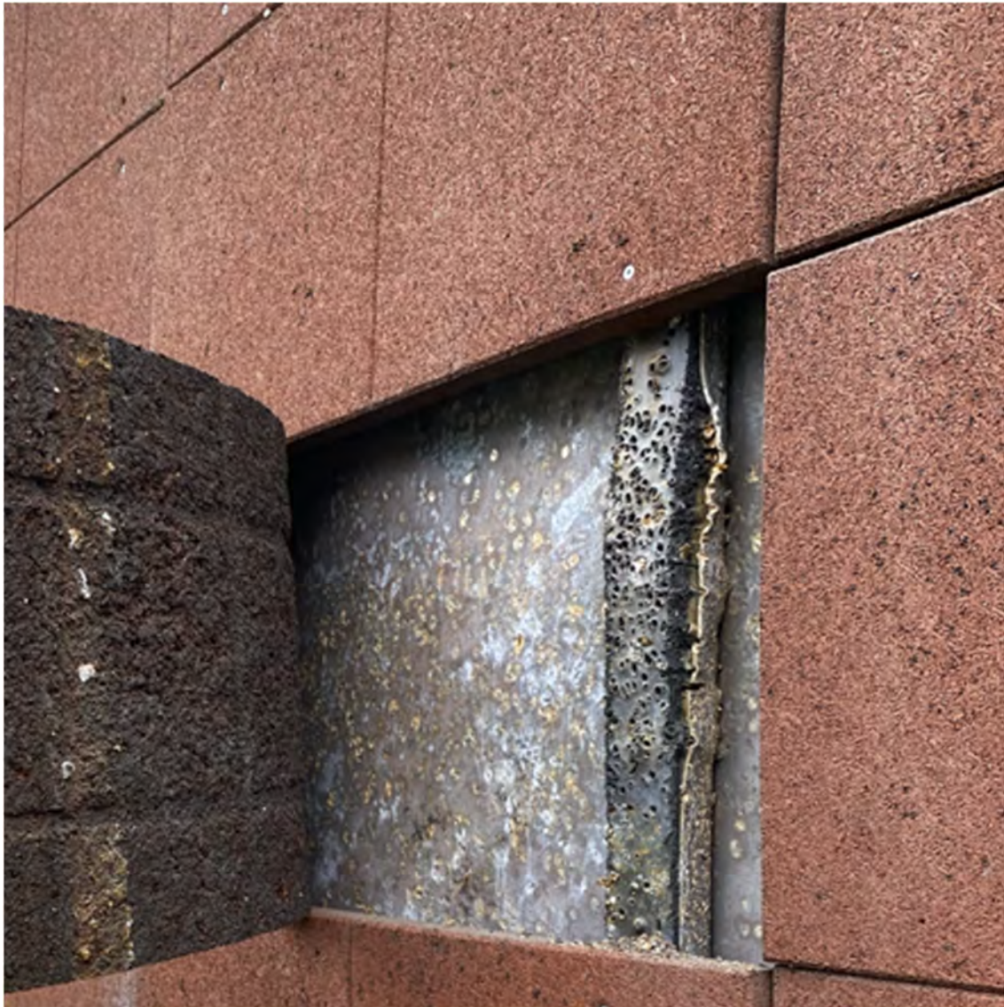
Figure 29 Picture showing the inside of the bullet trap on Range 10 at Sessvollmoen
