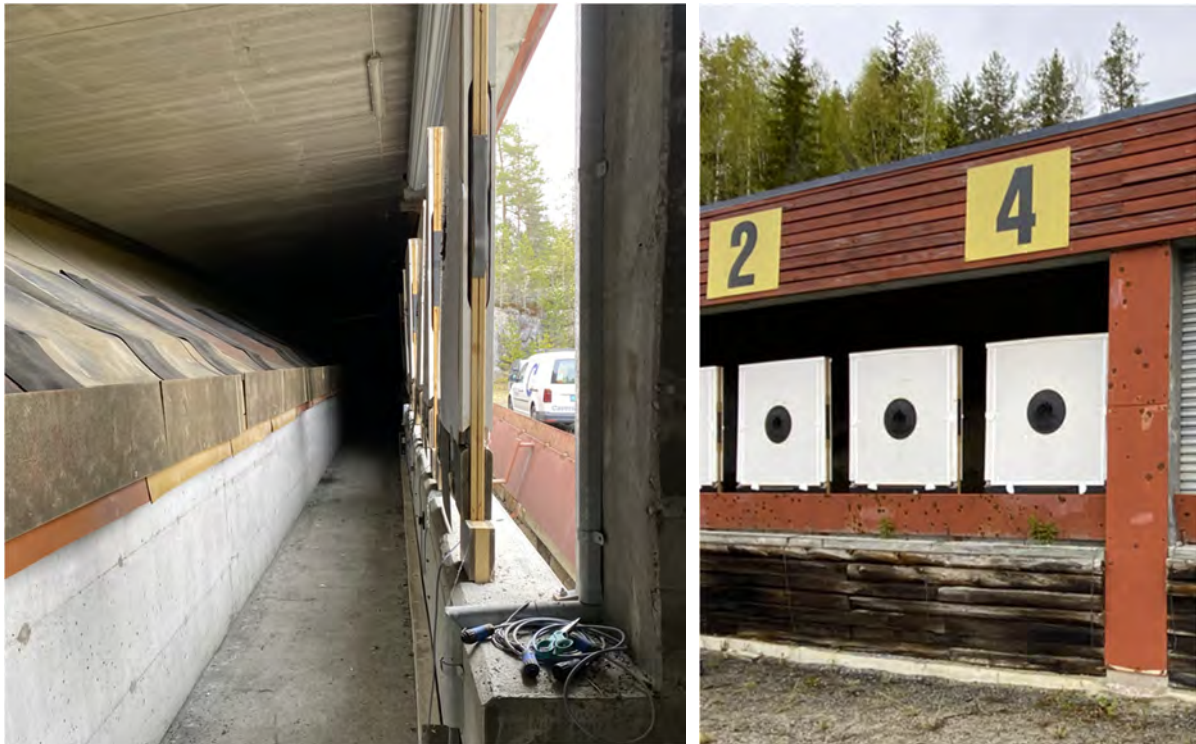
Figure 13 Sloped granular bullet trap with a cover and roof over it, at the Ringerike Gun Range
