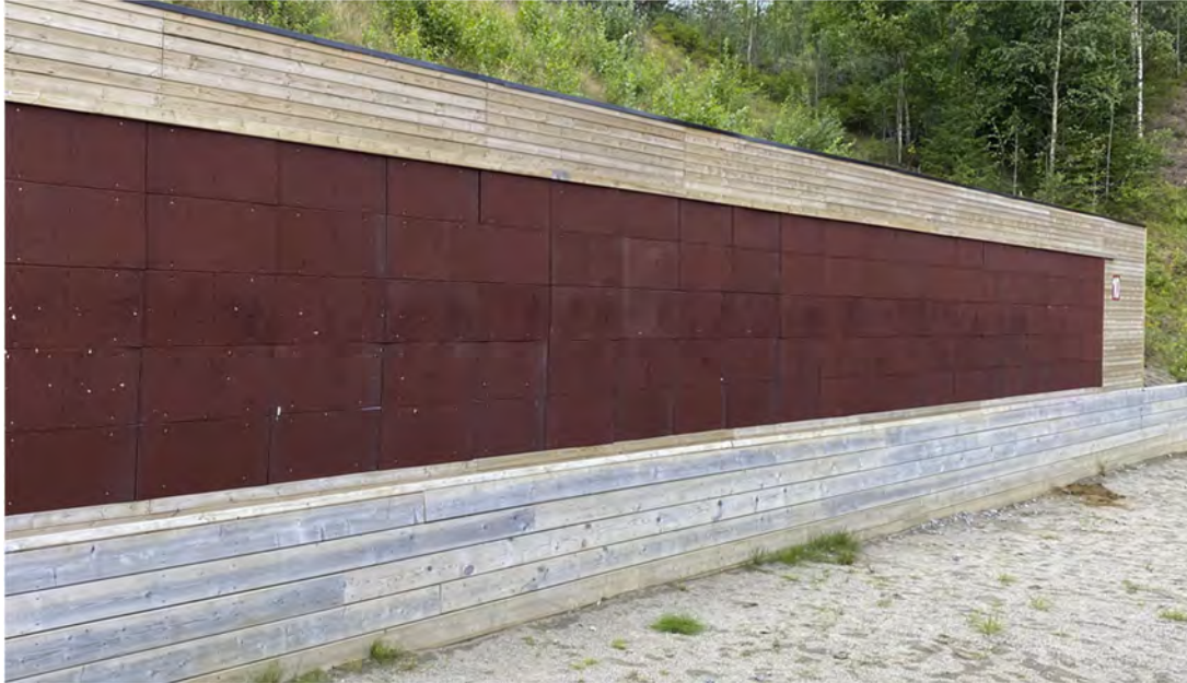
Figure 27 The bullet trap with a vertical steel plate on Range 10 at Sessvollmoen
