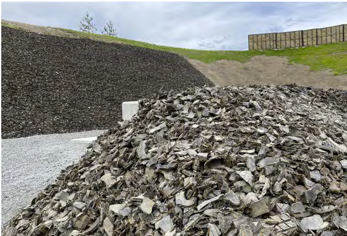
Figure 15 Target mound and bullet trap made of tyre chips, seen from the side
