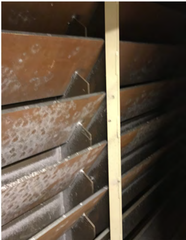
Figure 21 Steel lamellas in a bullet trap. The lamellas and the back plate are both made of Hardox steel plates
