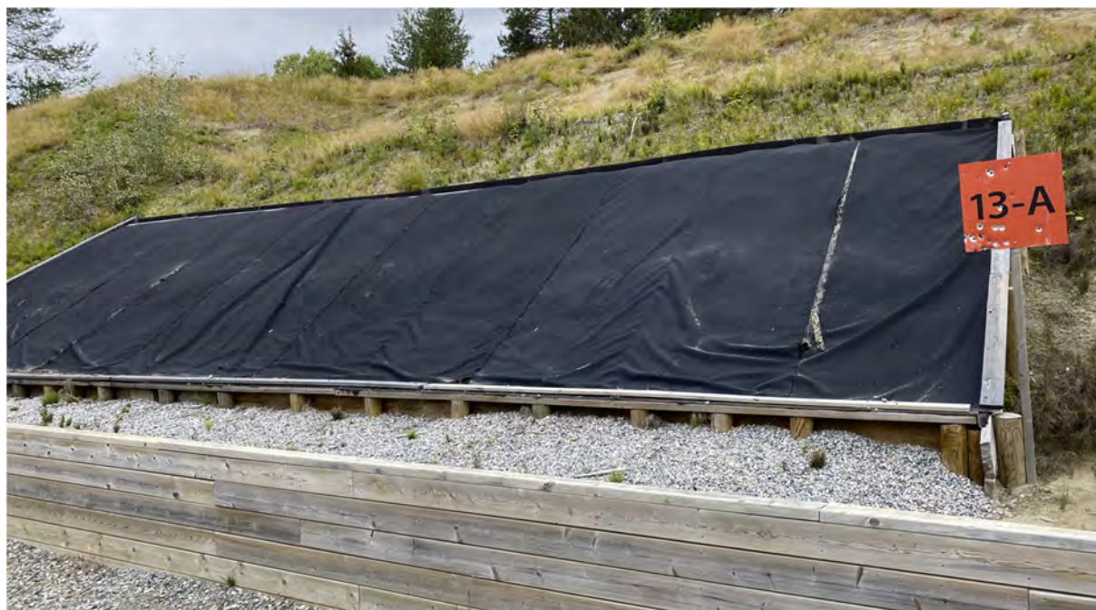
Figure 10 Granular bullet trap on range 13A at Sessvollmoen
